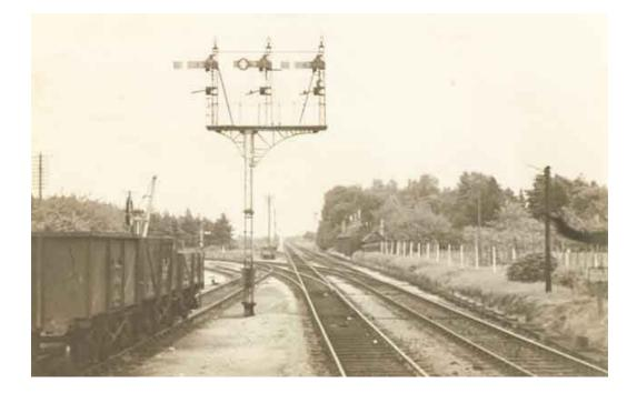
This view (above) shows the junction more clearly together with the iconic junction signals. The middle semaphore arm, with the circle attached, controlled traffic entering the MOD fuel depot sidings network. On the right of the tracks in the middle-distance can be seen the long line of single-storey 'railway cottages', dating from the middle part of the 19<sup>th</sup> century.
